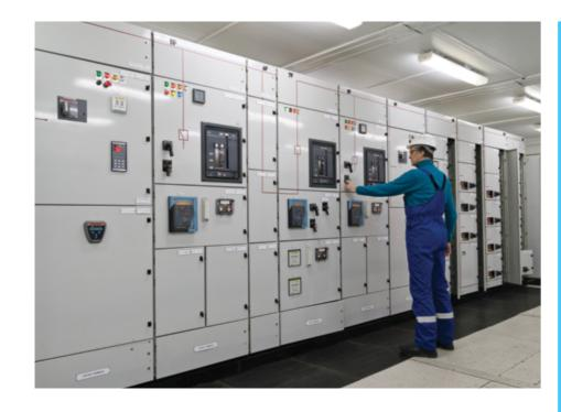
PCC panels upto 6300A have been built & supplied with one, two and three incomers.
